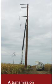
A transmission structure ready to be placed for the 161 kV line from the Chester substation.
