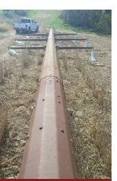
One of the transmission structures set in place for the 345 kV line coming from the Hampton substation.
