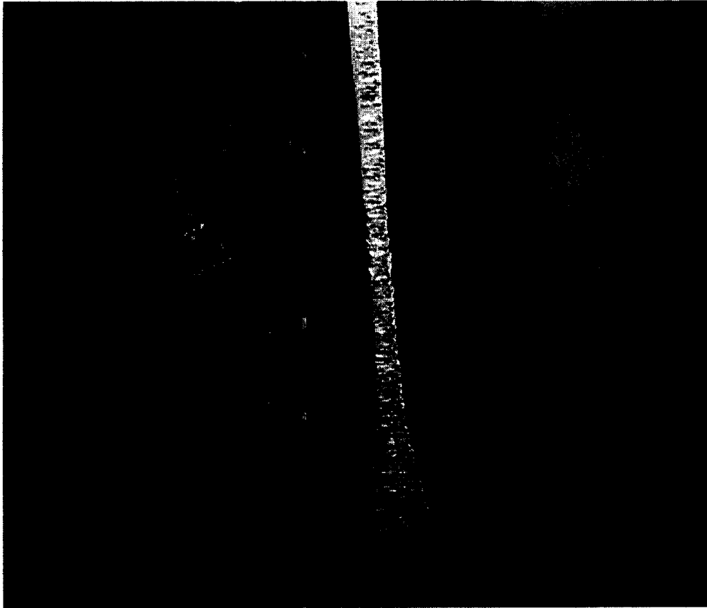
Figure 4 – Water particle impact damage to stage 17 bucket leading edge
