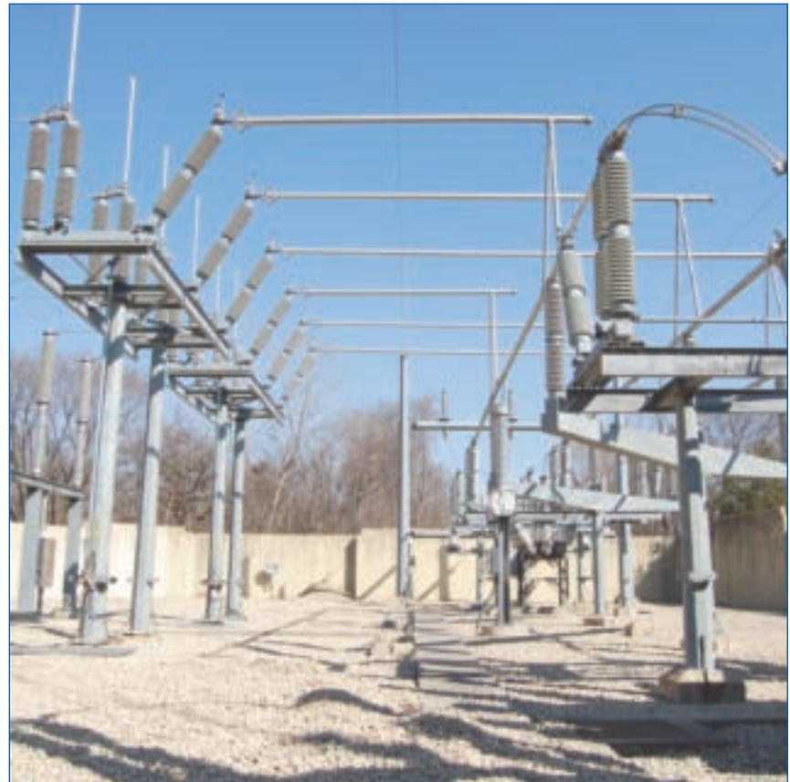
Bamber Valley Substation
