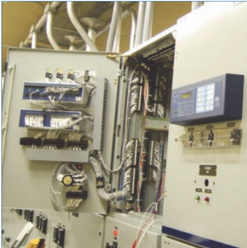
Protective relays inside the Bamber Valley Substation.
