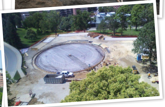
Steel rebars placed prior to pouring of replacement reservoir concrete floor.
