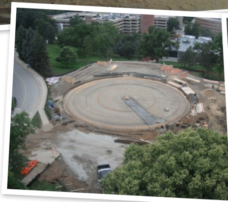
Concrete placed in forms to cast wall and dome panels.
