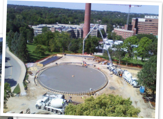
Pumping 250-yard continuous concrete pour of reservoir floor.
