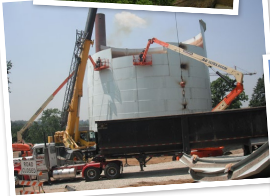
Old 1.5-million gallon reservoir being replaced by 3.3-million gallon reservoir.
