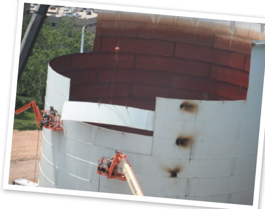
Demolition of old Saint Mary's Reservoir.
