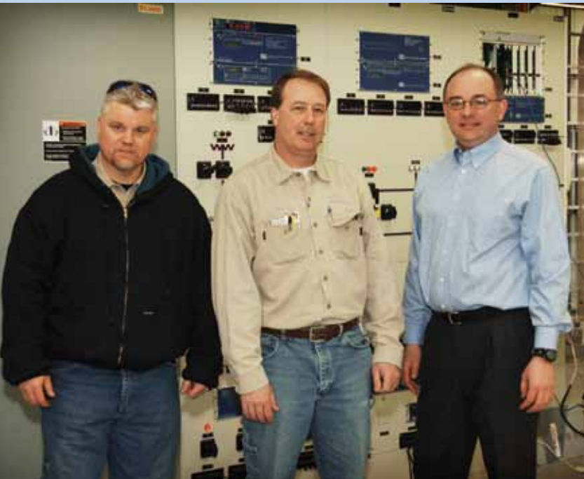
From left to right: Pete Minogue (Substation Electrician), Ted Mason (Utility Technician), and Neil Stiller at RPU's Westside substation. Substation staff not pictured are: Bill Schmitz (Substation Electrician) and Jeff Kranz (Lead Utility Technician).
